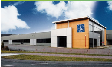
Hoogeveen (The Netherlands) Electronic Controls
