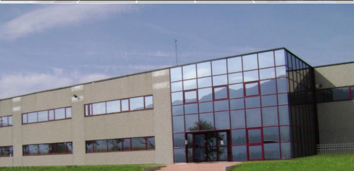
Brasov (Romania): Mechanical Controls, Integrated Systems, Fans, Gas Meters
