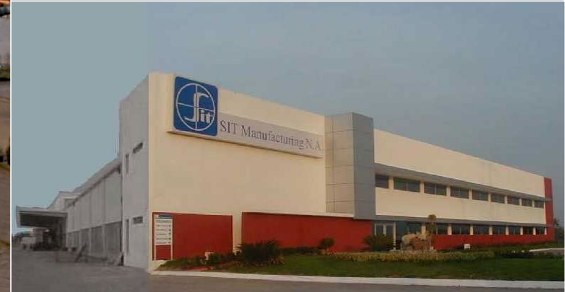
Monterrey (Mexico): Mechanical Controls, Sensors
