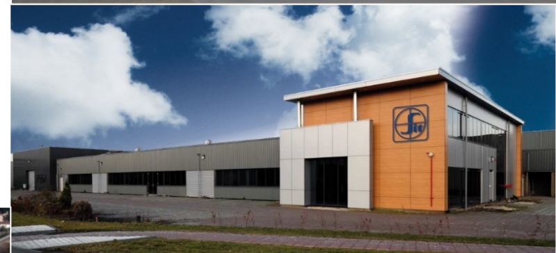
Hoogeveen (The Netherlands): Electronic Controls
