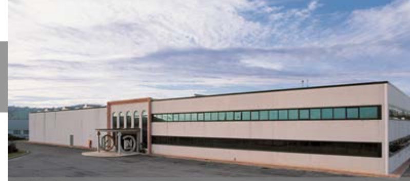
Montecassiano (Italy): Fans, Exhaust Systems
