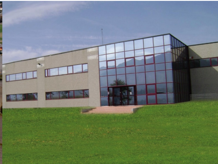
Brasov (Romania): Mechanical Controls, Integrated Systems, Gas Meters
