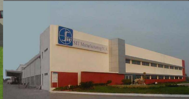
Monterrey (Mexico): Mechanical Controls, Sensors
