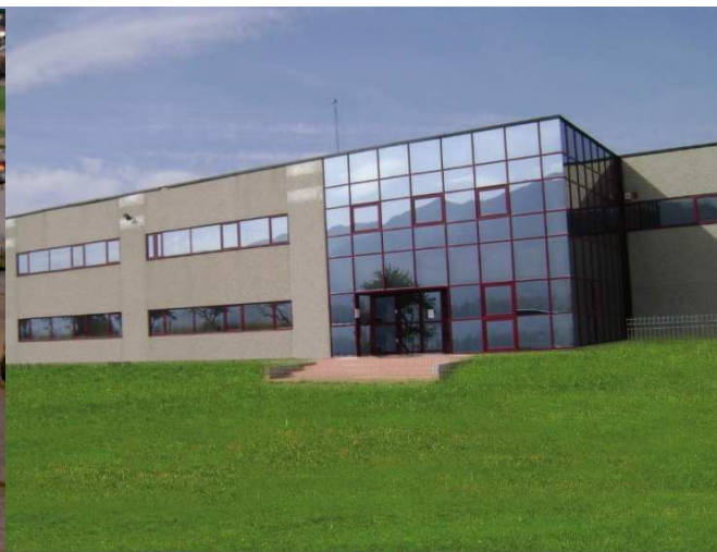
Brasov (Romania): Mechanical Controls, Integrated Systems, Gas Meters
