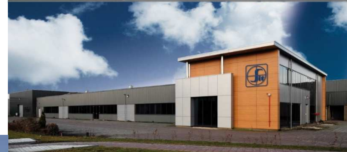
Hoogeveen (The Netherlands): Electronic Controls
