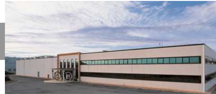
Montecassiano (Italy): Fans, Exhaust Systems
