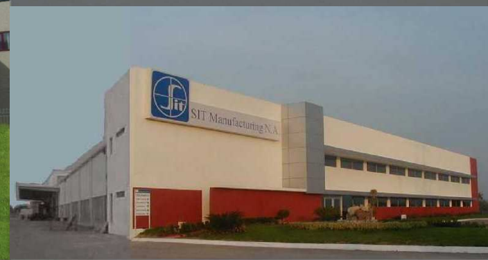
Monterrey (Mexico): Mechanical Controls, Sensors
