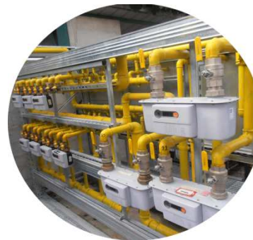
Smart Grids: Gas Metering
